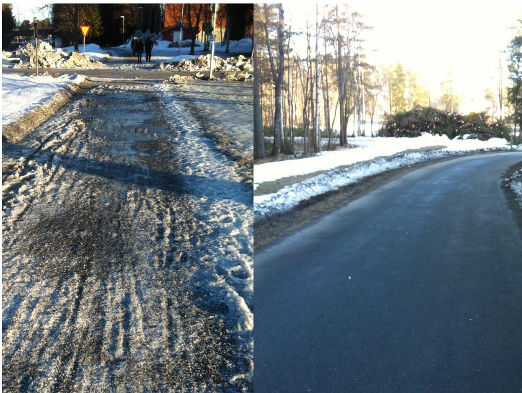
Figure 2C4. To the left is a cycle path on a sunny winter's day. Despite ploughing and spreading of sand the bicycle paths can become tracked and difficult to ride. To the right snow removal by sweeping and spreading road salt has been tested with a very satisfying result. The tests will continue during 2016.
